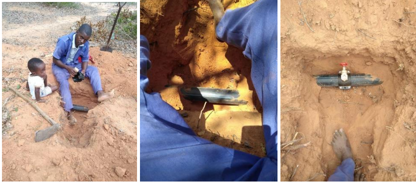
Figure 10. Connecting to the 3-inch main pipe
