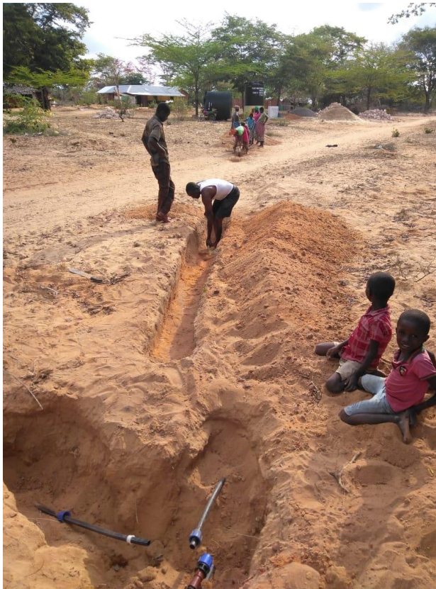
Figure 9. Trench digging and pipe laying.
