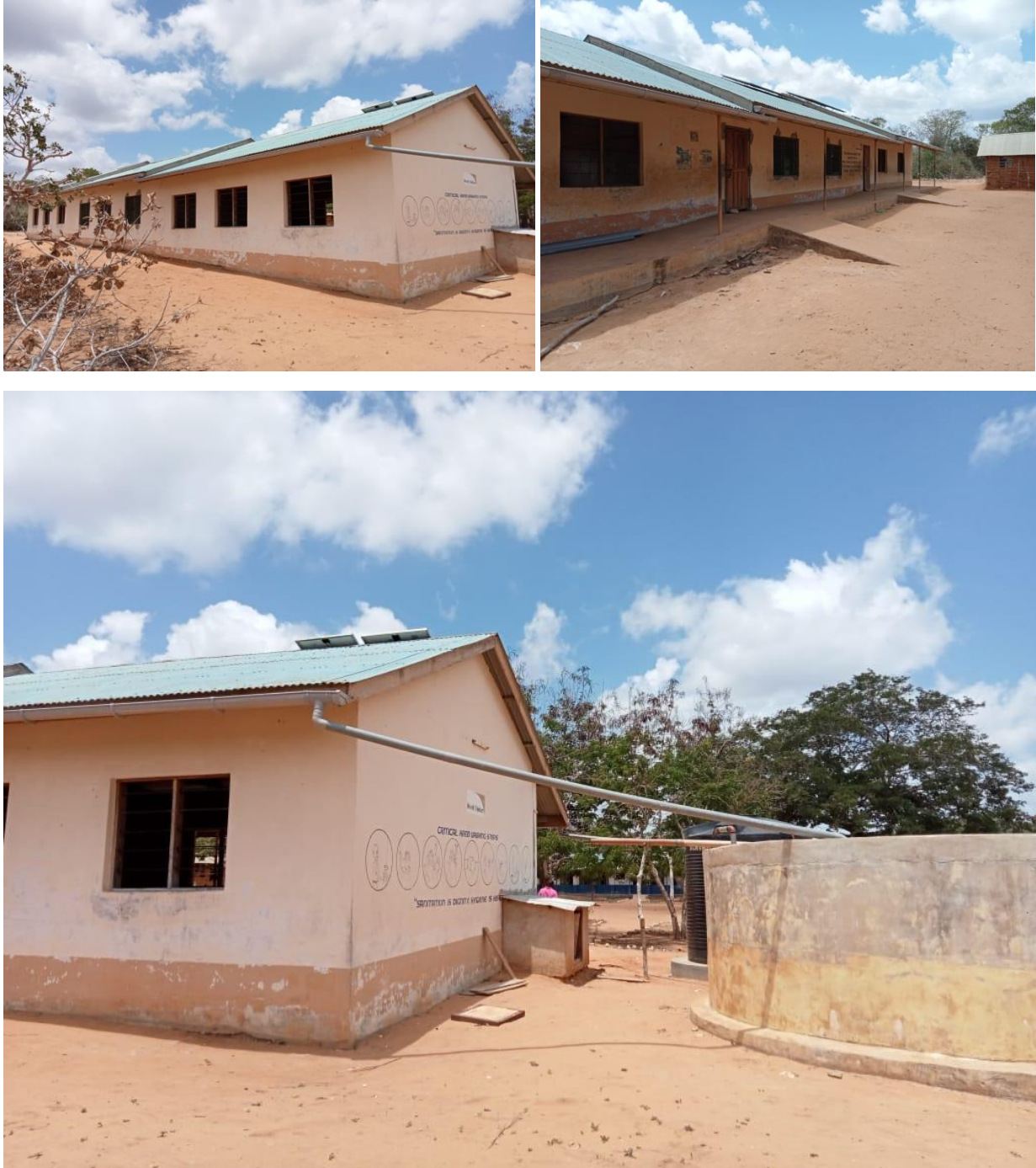
Figure 14. The gutter system is fully installed!
