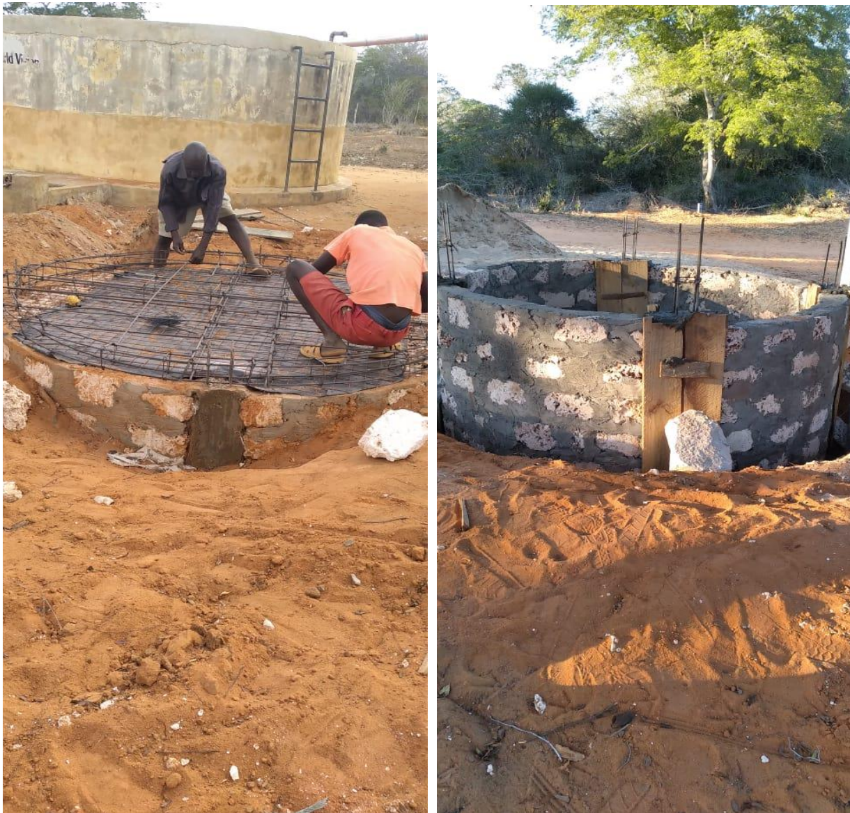
Figure 11. Concrete slab construction. At school and village.
