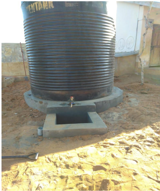
Figure 12. Slab completion and tank fitting.
